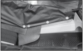
Fig 75 - Transition corner flashing in place
