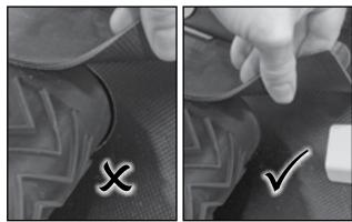
Fig 77 - Corner flashing must fit tight around the belt
