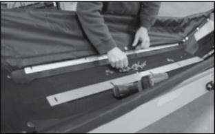
Fig 76 - Stainless steel flat bar to hold side flashing
